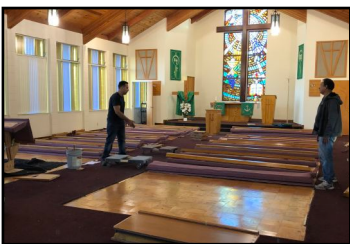
Pews Removed for Refurbishment, October 28, 2019
