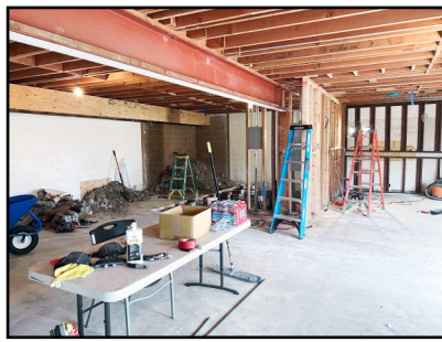
Fellowship Hall Remodel in Progress, June 3, 2022
