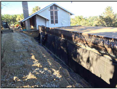
Classroom Building Excavation to Replace Failed Waterproofing, Summer 2016
